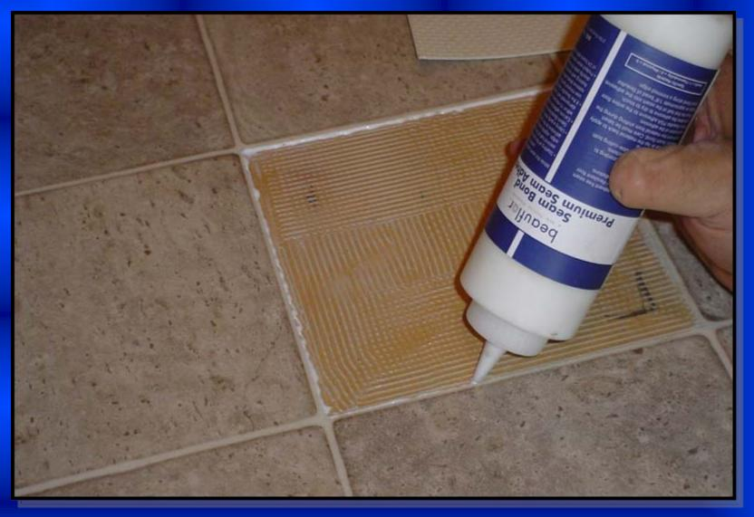
Apply an 1/8" bead of resilient flooring seam bond adhesive around the entire insert perimeter.
