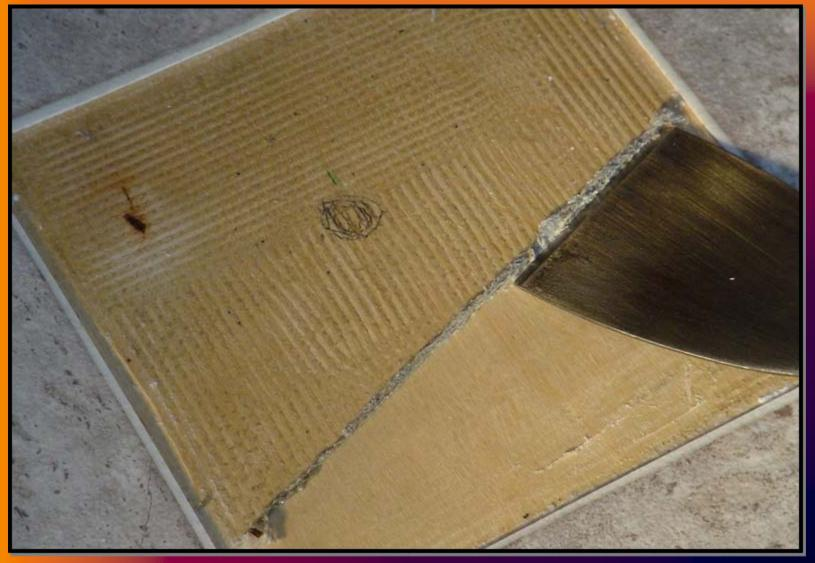
With a sharp scraper remove the adhesive down to a thin residue.
