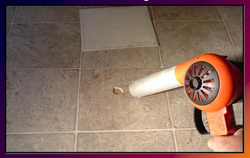
Completely heat the area to be removed until warm to touch to soften the adhesive beneath.
