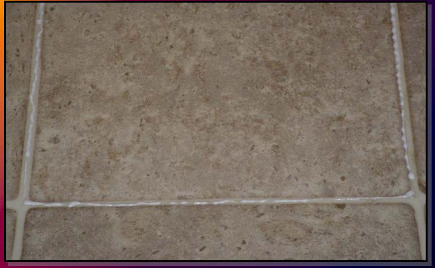
Carefully tuck the insert into place forcing the seam bond adhesive up into the seam.
