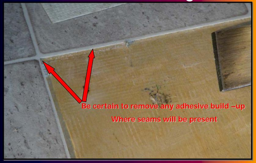
Carefully clean the adhesive along the seam and in the corners to prevent any seam "ledging".
