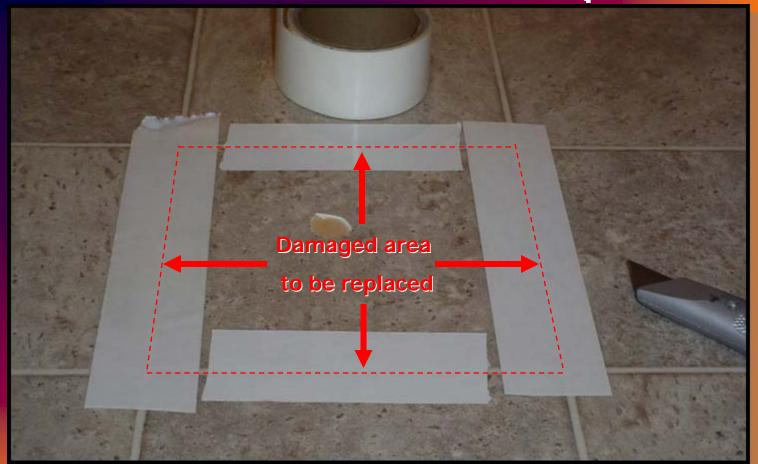
Position the tape where cuts will be made. Cuts should be made in grout lines or areas where the flooring pattern will camouflage patch edges.
